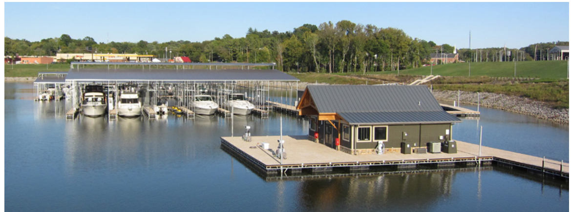
Floating docks and marina administration building, Clarksville, Tennessee
