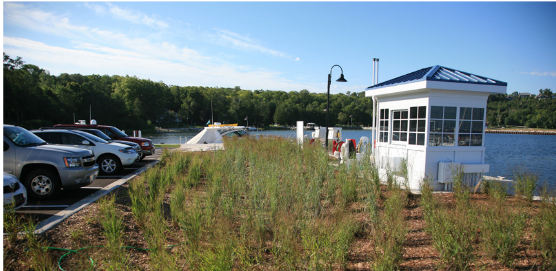
Vegetated stormwater buffer between the parking lot and harbor at Egg Harbor Marina
